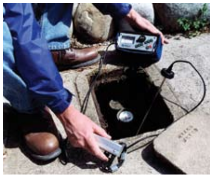
Leak Surveying by listening at a meter with contact rod
